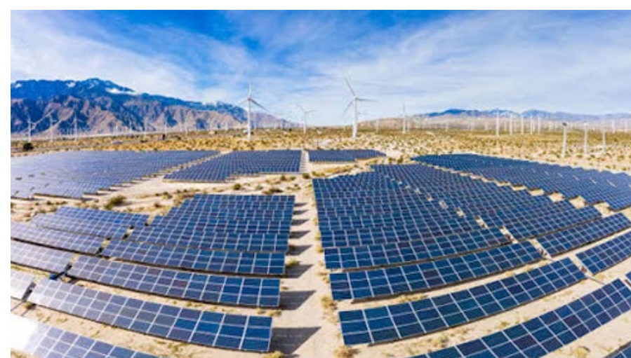
Figure 2: Battery energy storage systems are widely used in solar and wind farms. (Image source: Integra Sources LLC )
